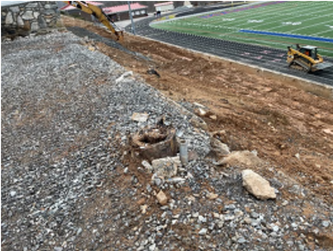
^ (E) old pine light pole, replaced by concrete poles
