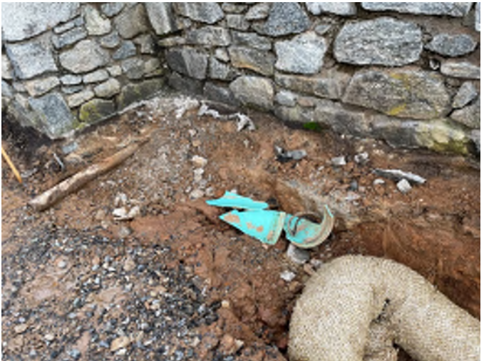
^ (E) upper concourse walk removed at (E) drain line
