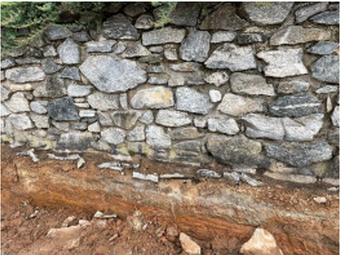
^ Existing granite wall and footing
