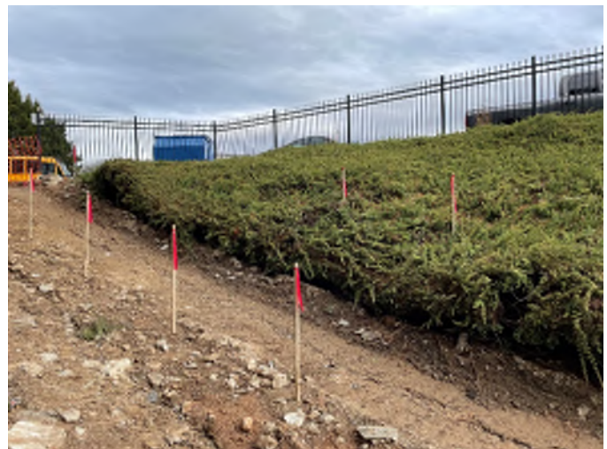
^ Portion of granite wall demolished.
