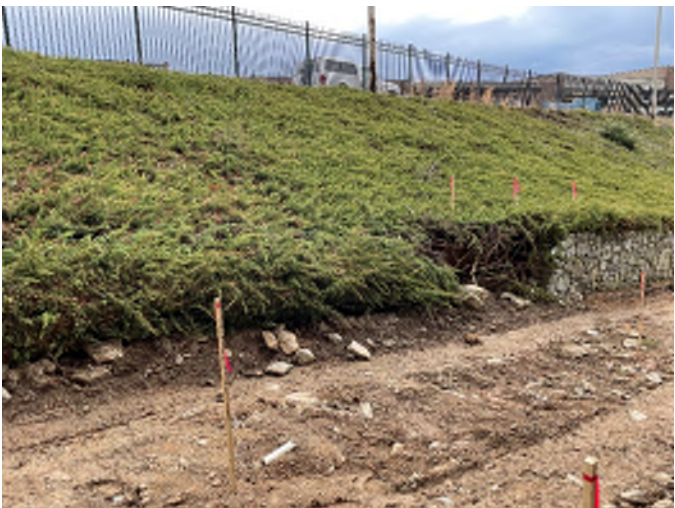
^ Portion of Granite wall demolished
