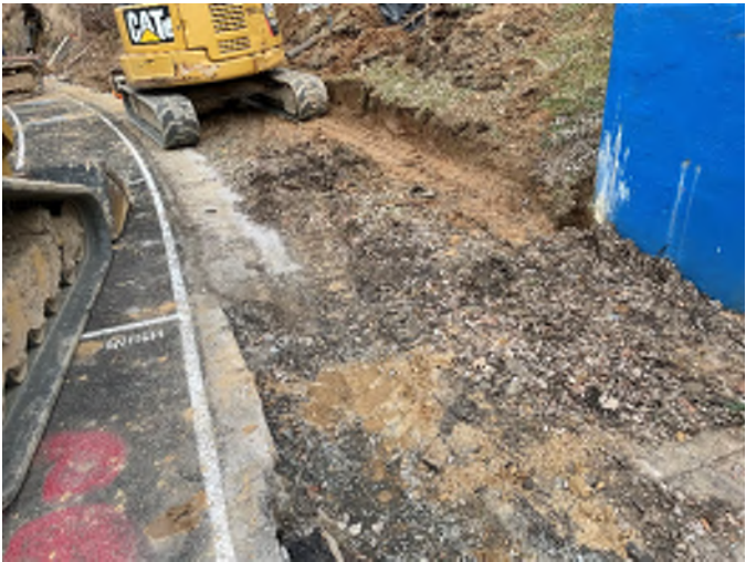
^ Existing lower sidewalk slab removed, east of stadium
