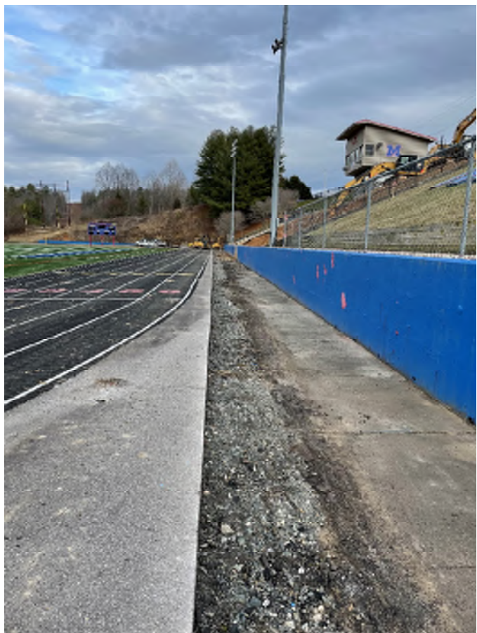
^ Saw cut made, existing sidewalk to be demo'd and replaced
