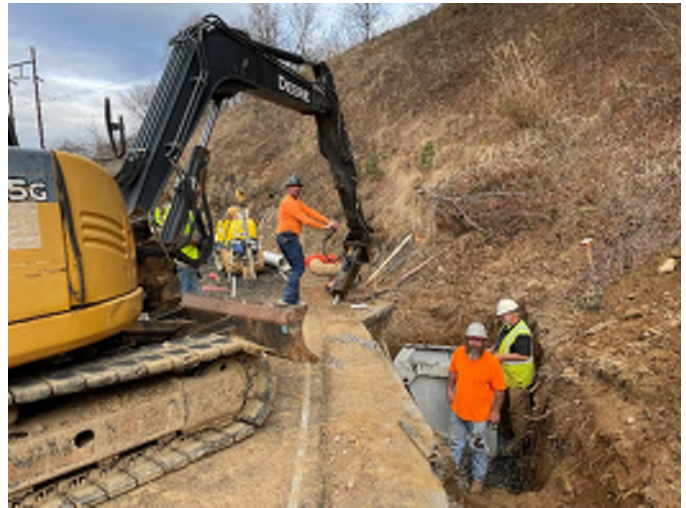
^ New drain box being installed at track level
