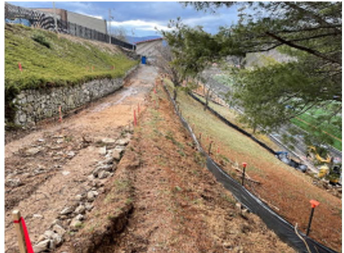
^ ADA ramp staked
