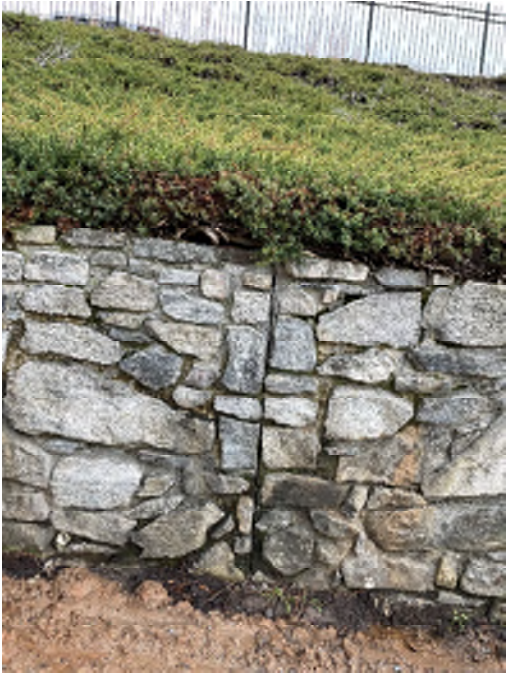
^ Granite wall existing control joint
